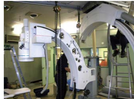
▲ The scene of dismantling and carrying out cerebral angiography device
