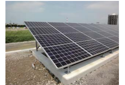
▲ KYUSHU ELECTRIC POWER CO., INC. Omuta mega solar power plant (3,000KW)
