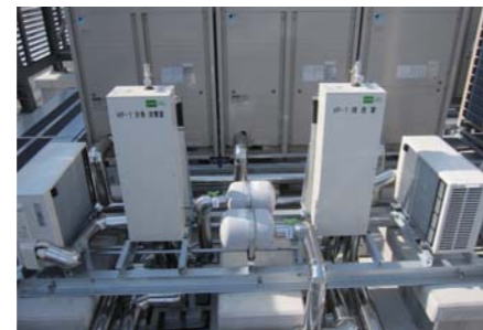
▲ High efficiency heat pump equipment
