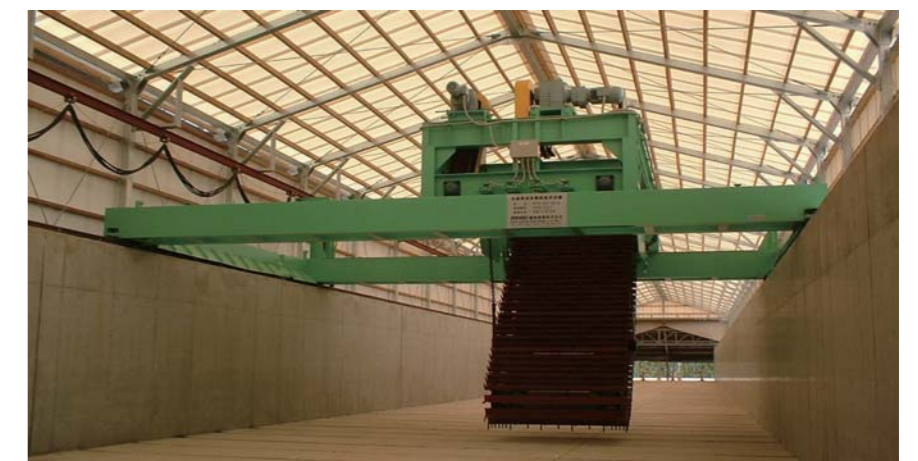
▲ 24 hours full automatic unmanned operation
