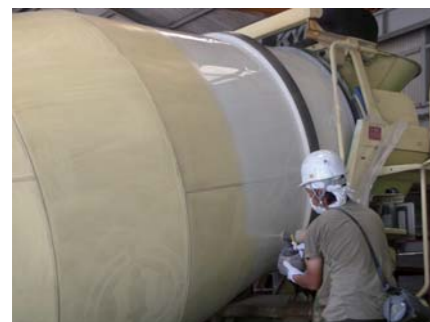
▲ Heat shield coating for ready-mixed concrete truck
