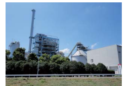
▲ Miyazaki Biomass recycled power generation plant
