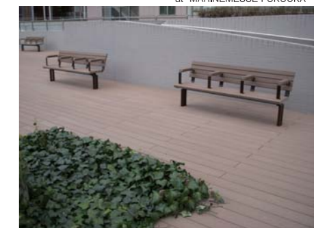
▲ An example of construction of deck and bench at "KYUSYU UNIVERSITY HOSPITAL"
