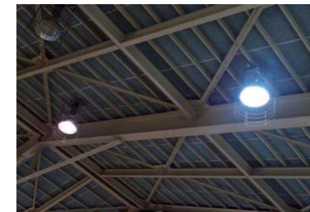
▲ (Left) mercury lamp 700W (Right) electrodeless lamp 250W
